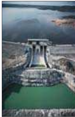
One of the vast power stations at James Bay
