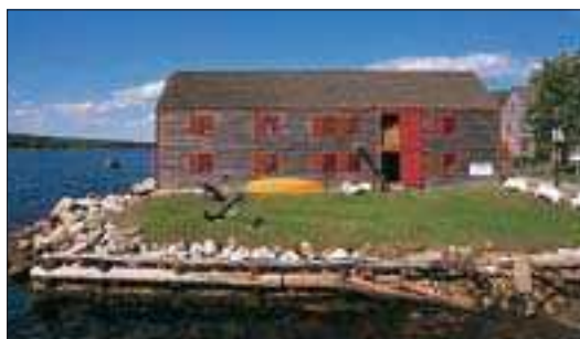
The Dory Shop Museum in Shelburne, center of local boat-building
