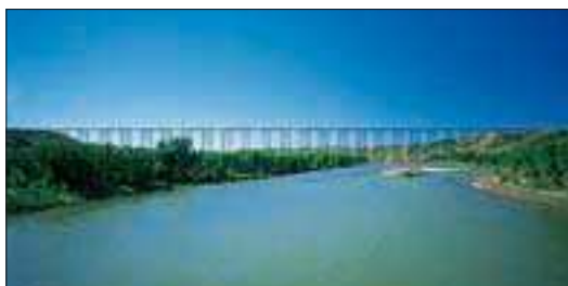
Iron Bridge over the Oldman River, Lethbridge
