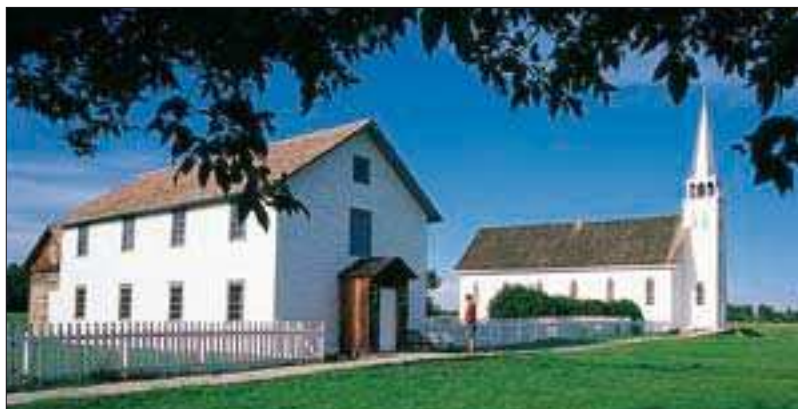
St. Antoine de Padou Church and Rectory at Batoche National Historic Park
